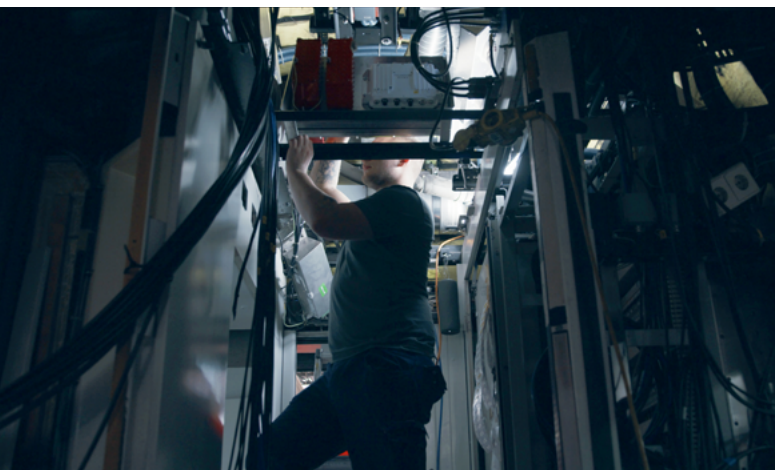
// DB employee installs Colibri
